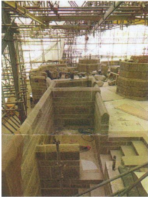
Parapets rebuilt on the central tower
