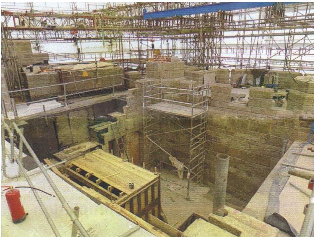
Central Tower Rebuild
